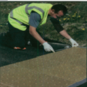
4 Applying duct tape
