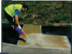
9 Broadcasting kiln dried sand
