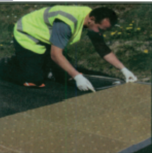
4 Applying duct tape
