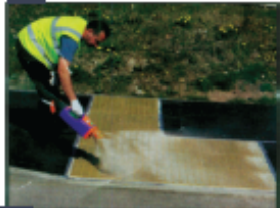
9 Broadcasting kiln dried sand
