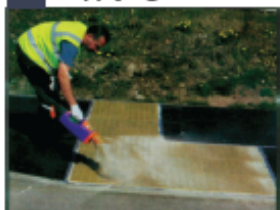
9 Broadcasting kiln dried sand
